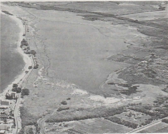
Kealia Pond, Maui, showing the existing aquaculture facilities on the right.
