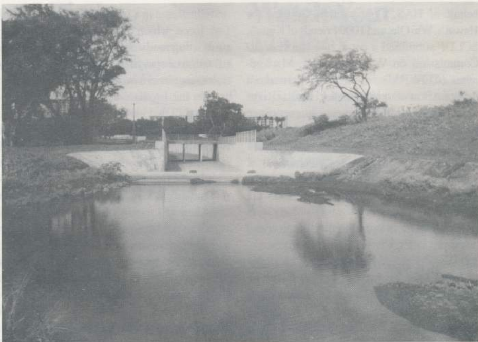
Desilting basin and channel at Honokowai Stream, Maui County's solution to sedimentation of nearshore waters.
