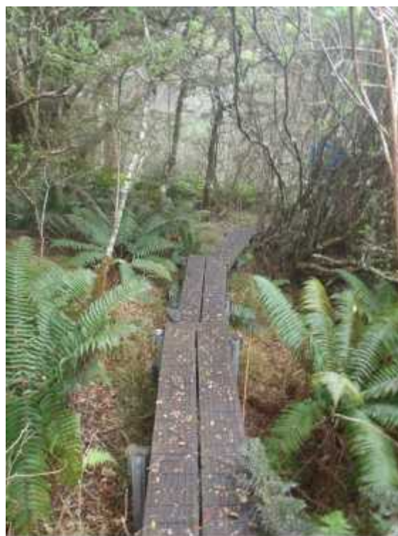
The boardwalk has no railings and a few places that are 2-3 feet off the ground, photo credit Colleen Soares.
